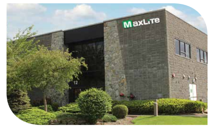
(HQ) West Caldwell, NJ
