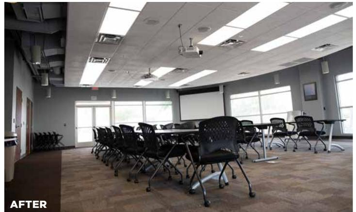
Utility wraps in the training and wellness rooms were retrofitted with MaxLite T5 lamps. The 67 existing two-lamp fixtures were converted from 28W fluorescent to the long-lasting benefits of LED via a simple ballast bypass.
