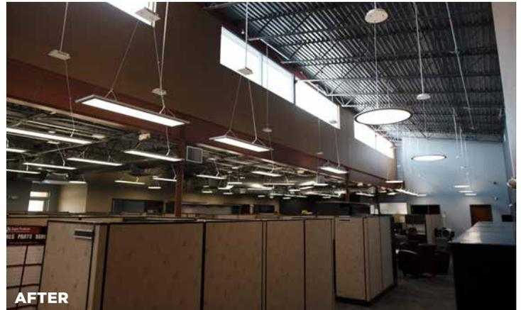
In the open office bullpen, employees complained of low light levels and shadows produced by the existing two-lamp indirect/direct fluorescent pendants. By applying a combination of MaxLite LED Indirect/Direct 1'x4' pendants and 2'x4' round pendants, Red Mountain was able to reduce the fixture count (from 73 to 64) and increase lumens to bring much-needed functional light to work areas. The slim form factors of the pendants also contributed to a more open and airy space.
