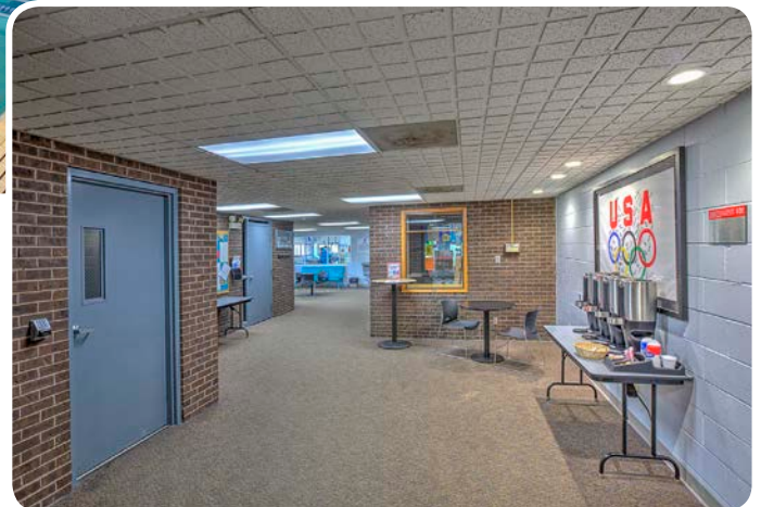
More than 600 18-watt LED T8 lamps, 14-watt recessed downlight retrofits and 10- to 16-watt omnidirectional A-lamps were used to replace fluorescent and metal halide bulbs throughout the facility. (Scott Evers Photography)
