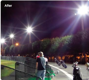
MaxLite's lighting applications engineering and design team developed a lighting plan using 48 270-watt and four 405-watt StaxMAX Floods that would provide more light while using less energy than the 78 existing 1,000-watt metal halide area lights, which consume 1,200 watts with the ballast.
